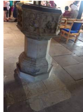
Moved Altar in small Chapel, and to the right, the font with the stone cut away to reduce falls and increase access.
